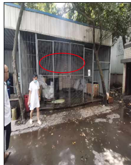
✘ 废料间未密闭, 且无废气收集设备
